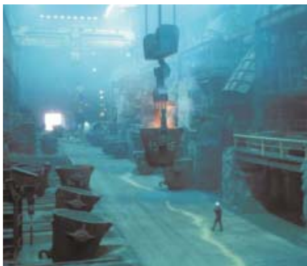
Inside the Nিকেleviy Zavod nickel processing plant, Russian Federation.
